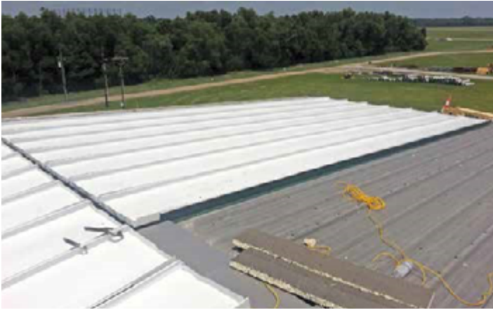
Figure 6 – Installation of the 24-gauge Galvalume symmetrical panels.
