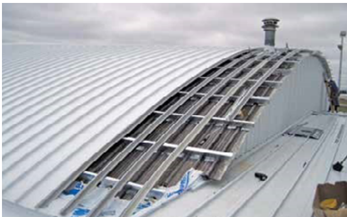
Figure 4 – Here, a 5-in.-tall Roof Hugger retrofit purlin and a 130-ft.-long curved symmetrical panel with 100% curved continuous clips were used to solve the problems of wind uplift and leaky transition.
